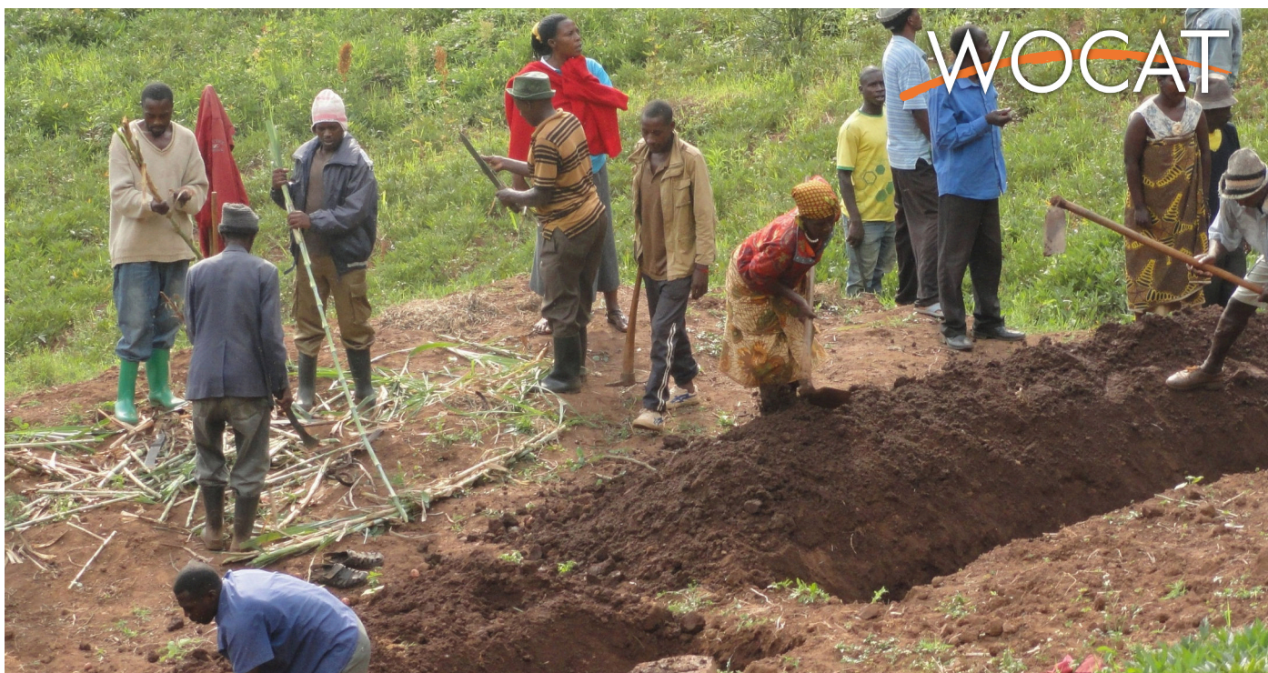
Excavation of soil and water conservation channels separated by tie bands (Kenneth Twinamasiko)
