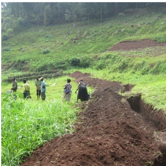
Excavation of soil and water conservation channels separated by tie bands (Kenneth Twinamasiko)
