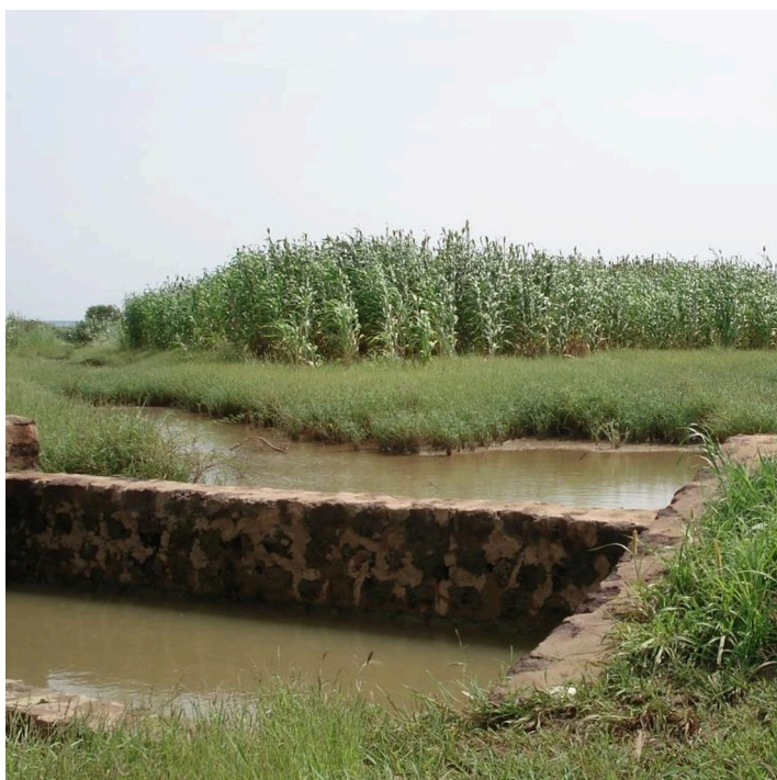
Water-spreading diversion weir during the rainy season (Heinz Bender)
