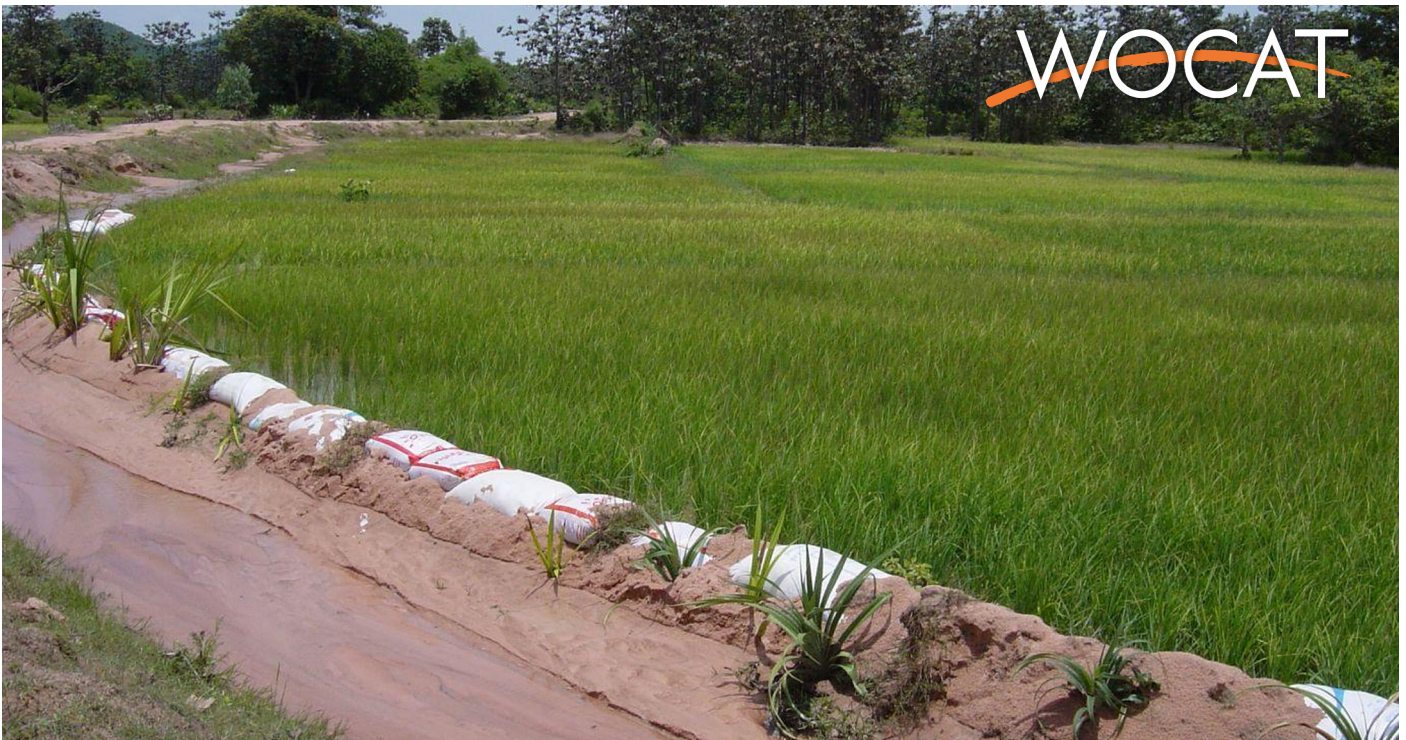
Recently stabilised dike with old rice bags and Pandanus, next to an irrigation channel and an eroding sand road. (Stefan Graf)
