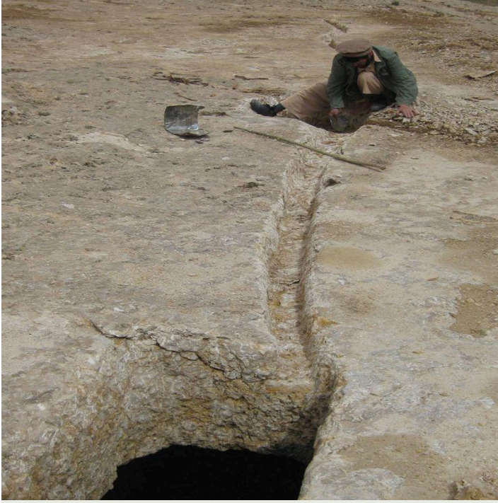
A view of the Kanda underground tank, conveyance channel, sediment pit (being cleaned) and the rocky catchment. (Helvetas Swiss Intercooperatio (Kabul Afghanistan))
