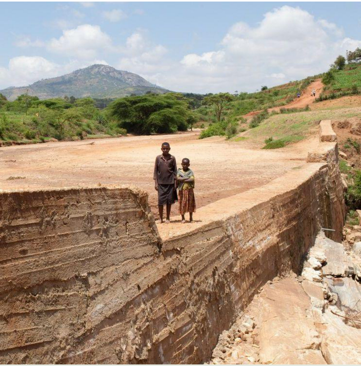
An example of a second mature sand dam in the same valley (Polly Braden (Daily Telegraph, London, UK))
