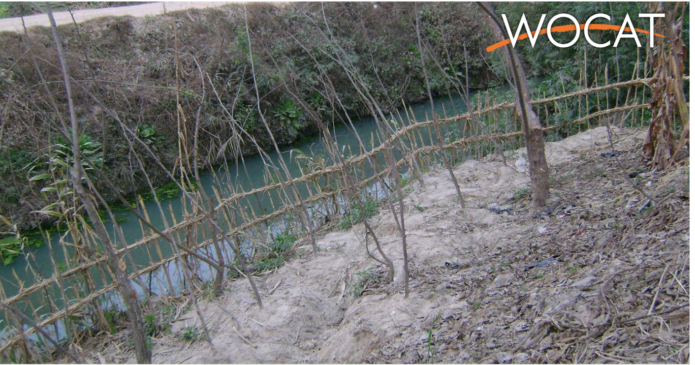
Newly planted Salix cuttings along the stream bank are protected by biofencing. (Indira Mulepati)
