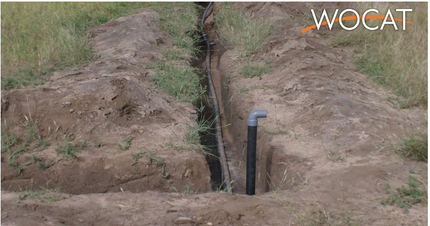
Pipes for the distribution of irrigation water are buried in 0.5 m deep canals (Sourakata Bangoura (Land and Water Resources Officer for Central Africa, Libreville, Gabon))
