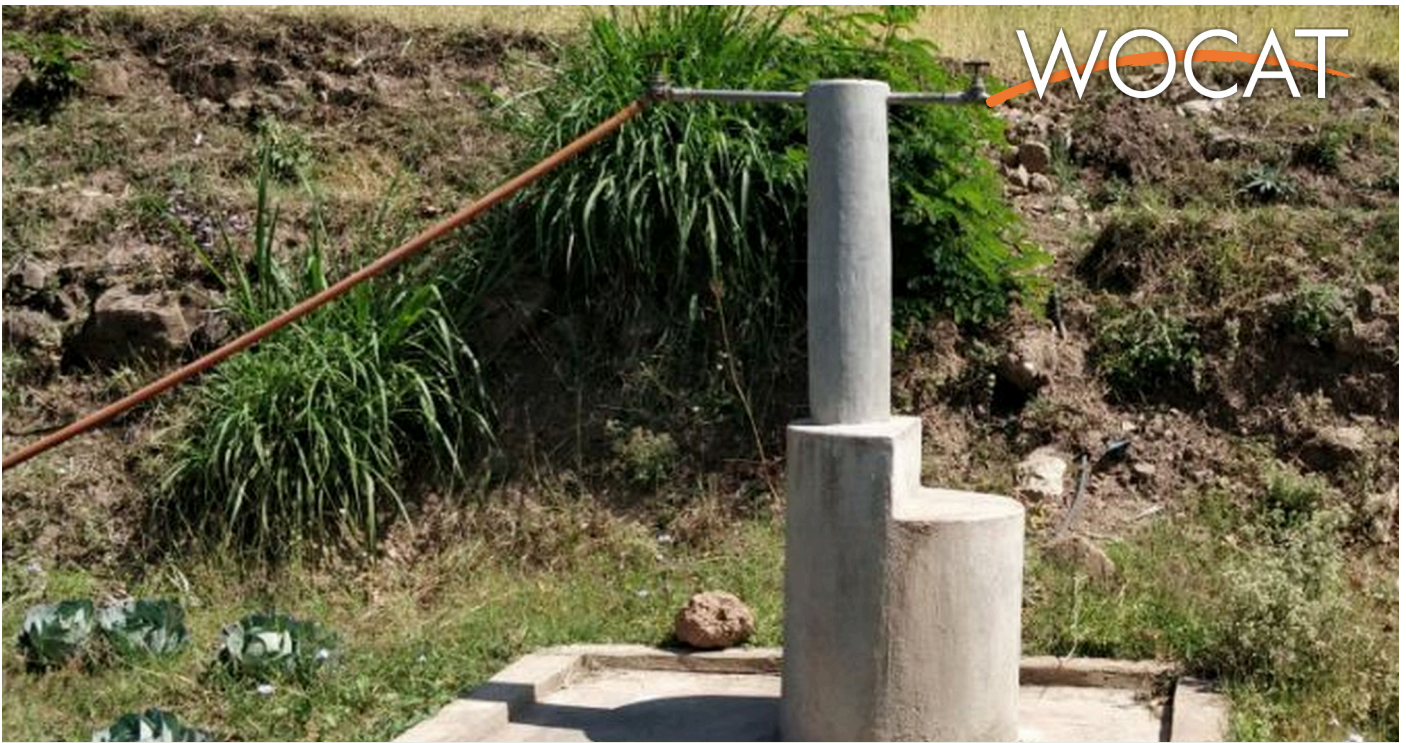
A MUWS Tower ("Thaado") with two faucets:- the one with pipe connected serves for irrigation and vegetable farming; the next faucet is for supply of drinking water. (Jhuna Kattel)
