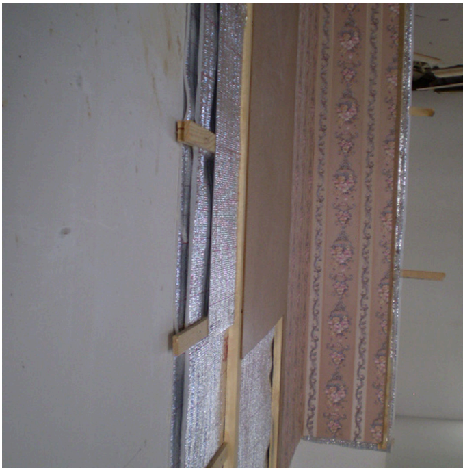
Thermo insulation of room by using foil (Zevارشoev Askarsho)
