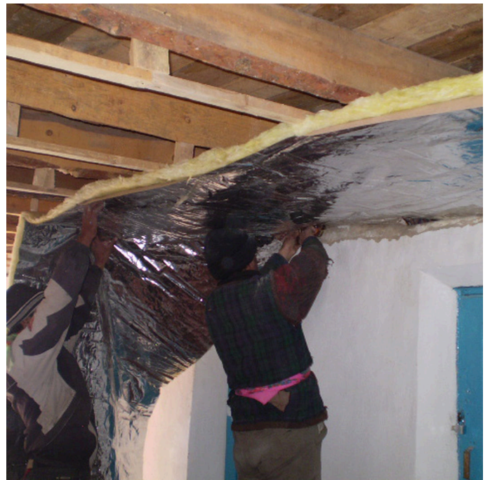
Training for local masters on thermo-insulation of ceiling (Khujamyor Khumorikov)
