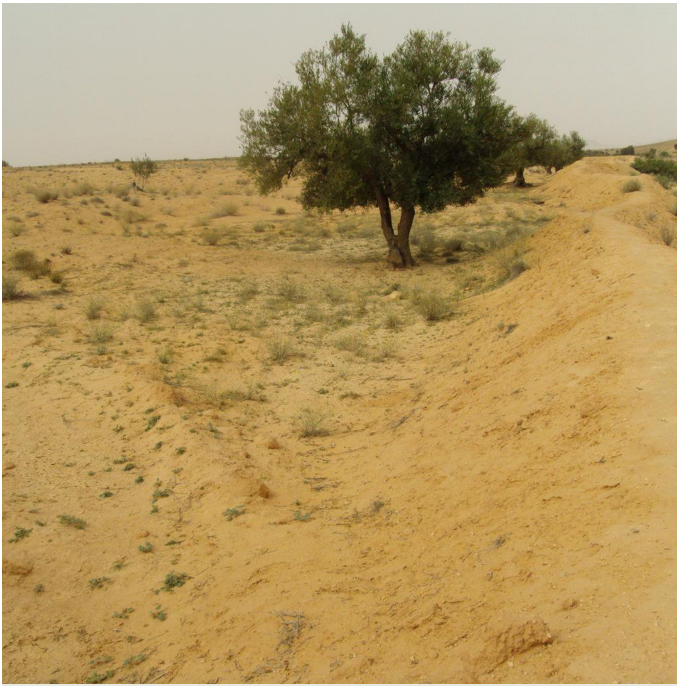
Tabia earthen dam in the Jeffara plain. Olive trees are generally grown along the dam, where the harvested water better infiltrates (Cyprien Hauser (WOCAT Bern, Switzerland))
