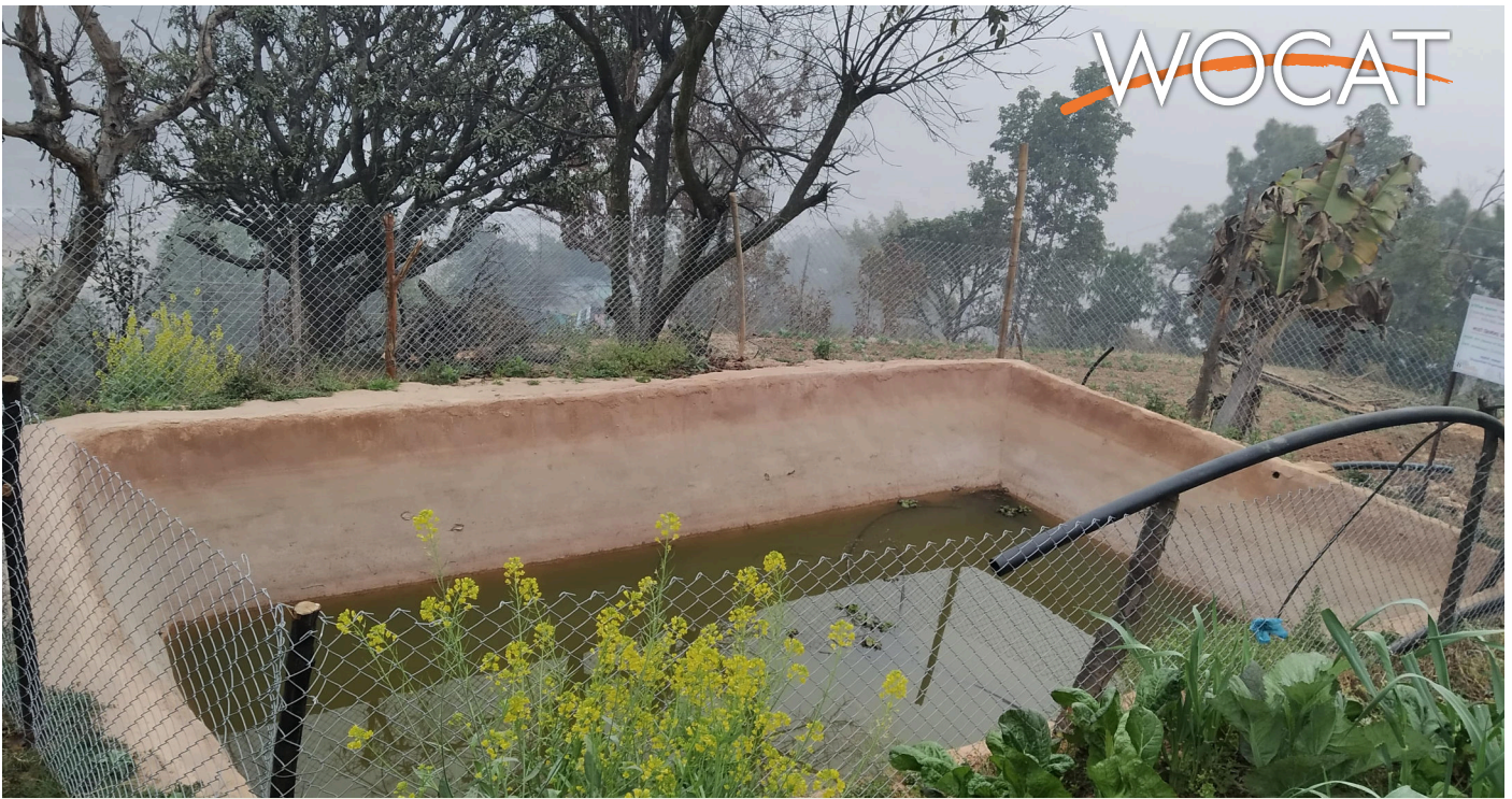
Soil cement pond of length= 7m, width= 5m and depth= 2m respectively (Kabita Nhemhafuki, ICIMOD)
