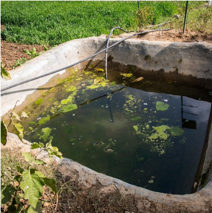
Soil Cement Pond of 4m length, 2m width and 1.5 m depth (Jitendra Bajracharya, ICIMOD)
