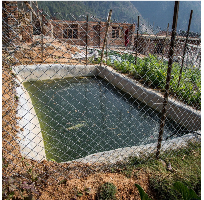
Soil Cement Pond of length 4m, width 3m and depth 2m (Jitendra Bajracharya, ICIMOD)
