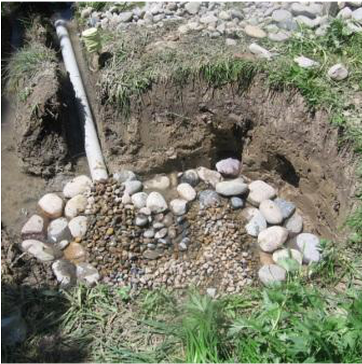
Positoning gravel on top of the perforated pipes. (Giuseppe Bonaty (CESVI))
