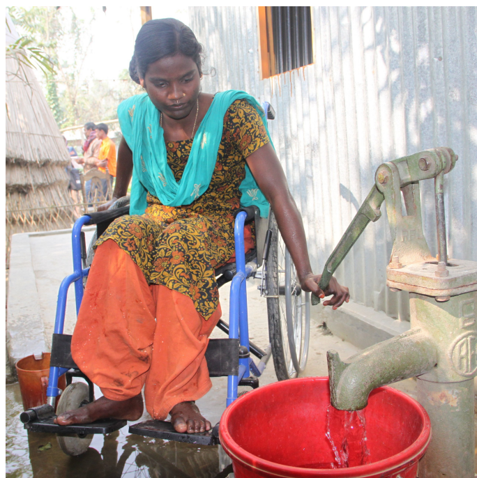
A women with disability using an accessible handpump wich was installed following the standards of universal design (Shahidul Islam, CDD)
