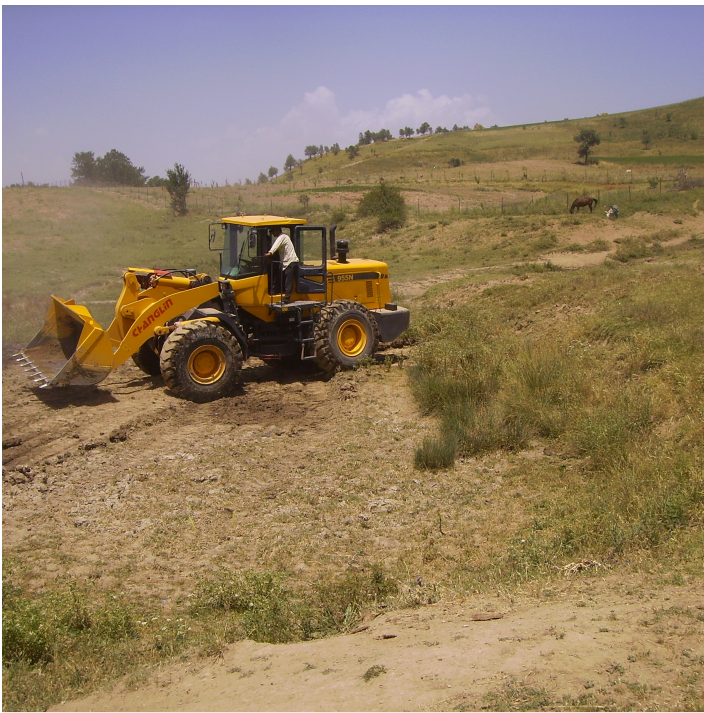
Pasture road rehabilitation (Toirov Safar)
