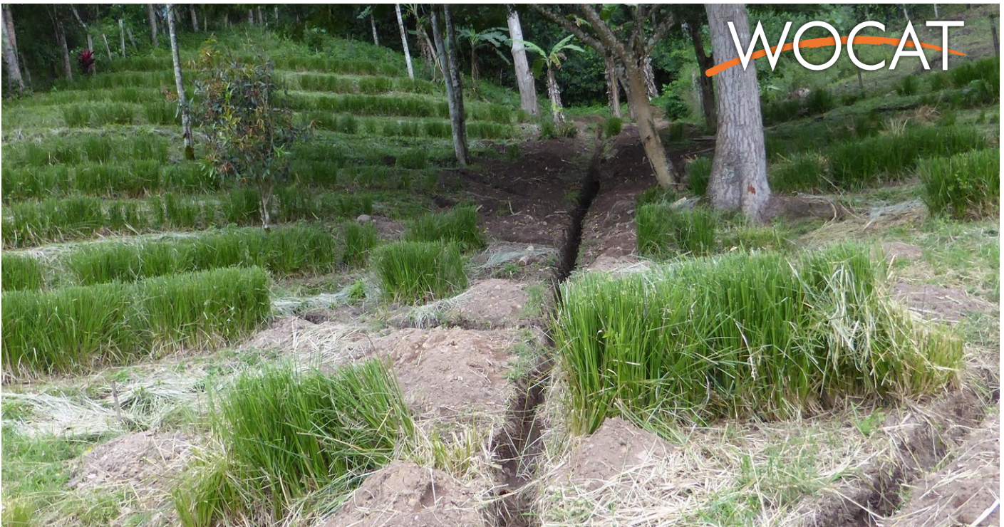
Fishbone shaped trenches waiting to be filled with fascine bundles before being covered with soil. (Helen Gambon, Swiss Red Cross)
