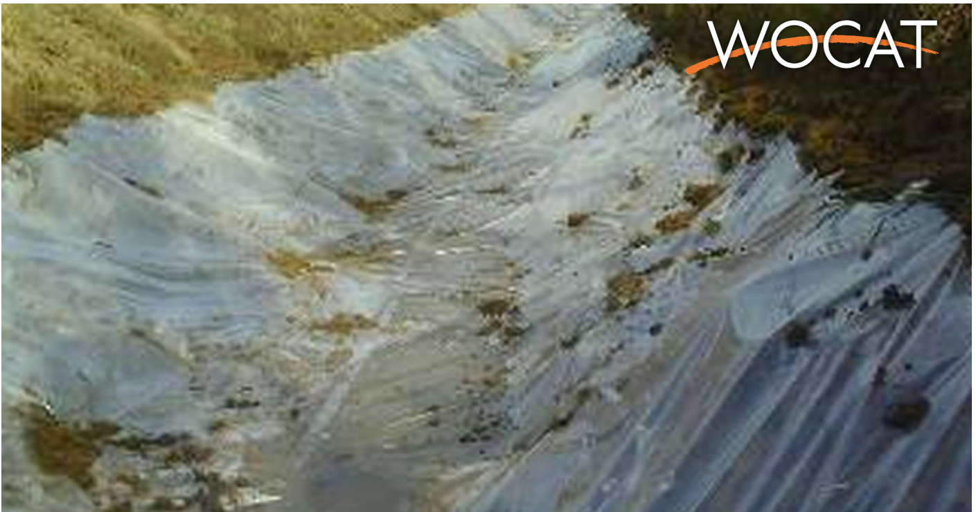
Laying of polyethylene film (Eshchanov R.A.)
