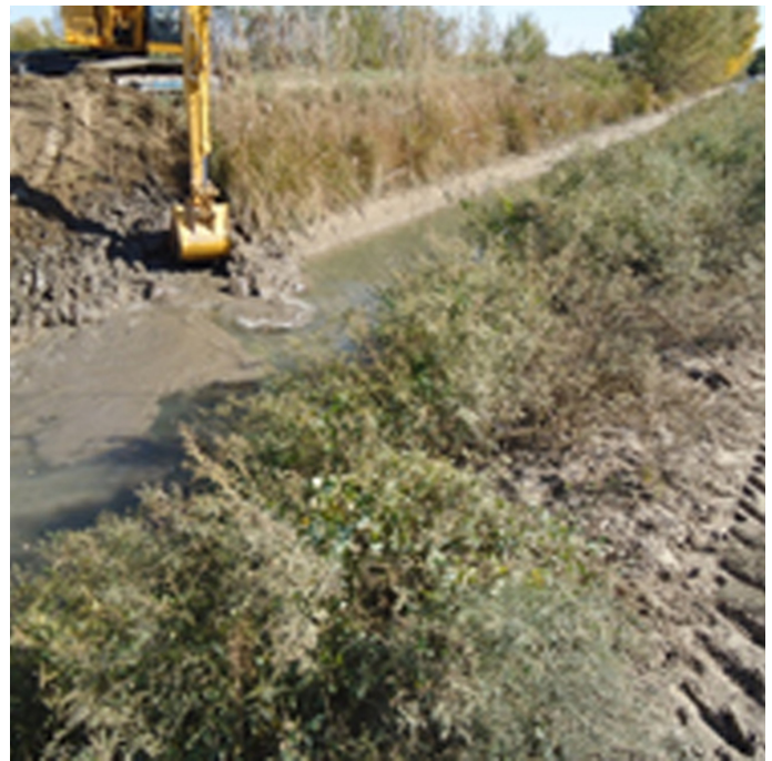
Channel cleaning (Eshchanov R.A.)
