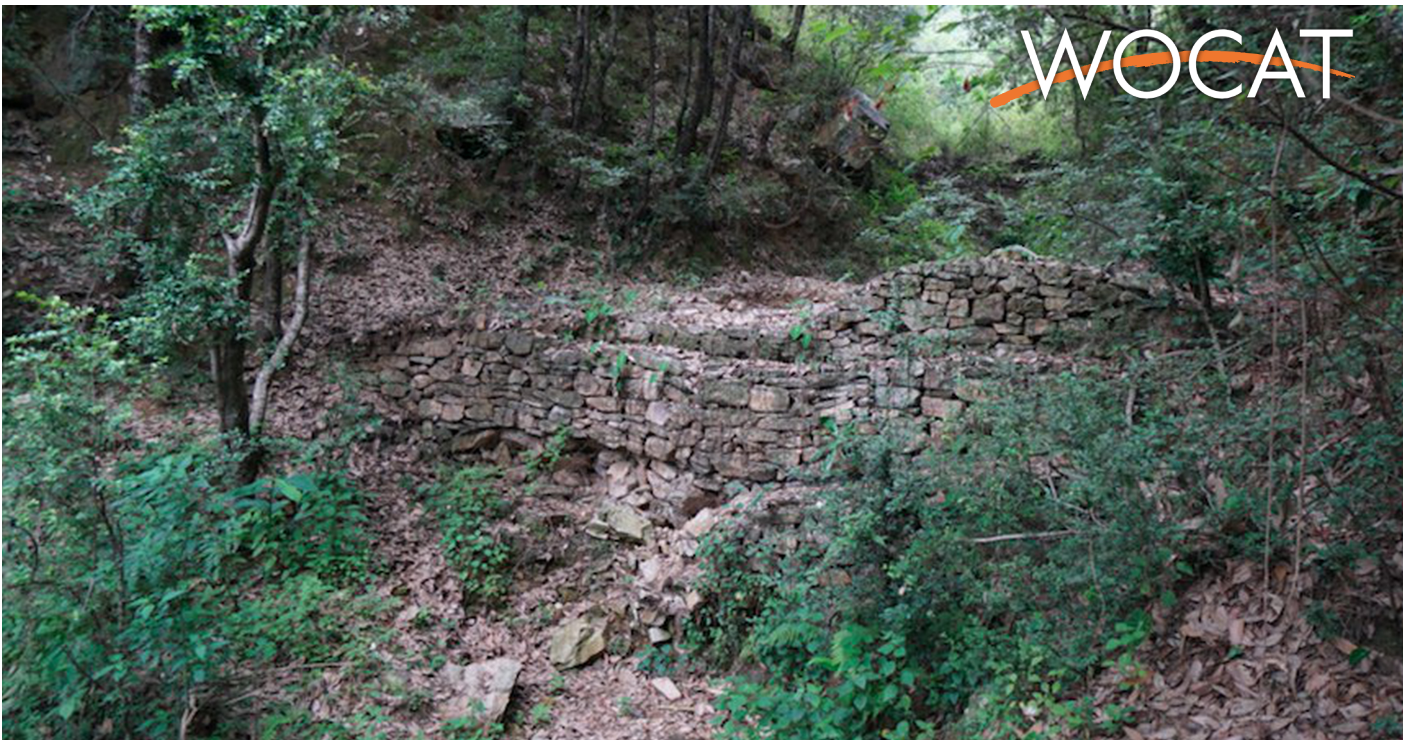
Stone Check Wall in Nakina Village (Hanspeter Liniger)
