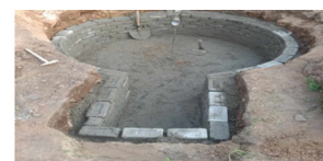
Digester where decomposition and production of methane gas occurs
