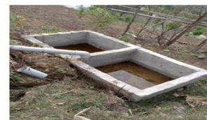
Slurry pit slurry that comes out of digester
