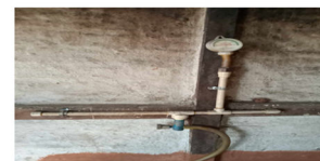
Pressure valve to check pressure of incoming gas from digester
