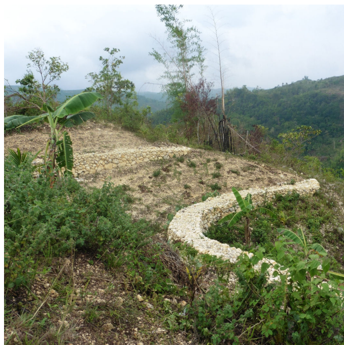
Rockwall built using the rocks available in the area (Engr. Djolly Ma. P. Dinamling)
