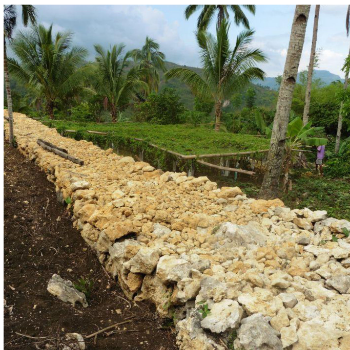
Rocks piled along contours. (Engr. Djolly Ma. P. Dinamling (Bureau of Soils and Water Management))
