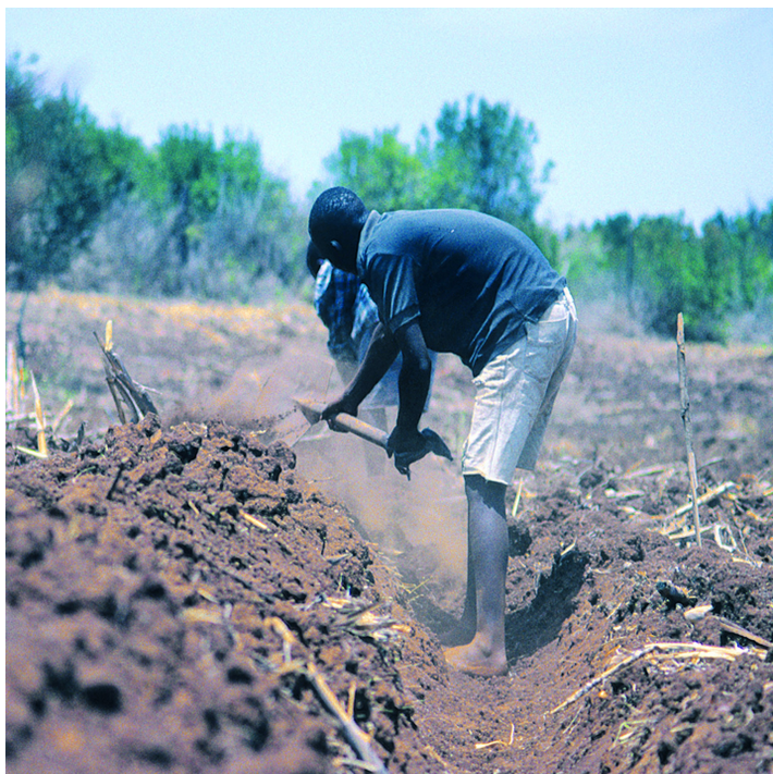
Construction of fanya juu terraces is heavy work. The name fanya juu means 'throw it up' in Swahili and refers to the first step of establishment: ditches are excavated and the soil is thrown upslope to form an embankment (Hanspeter Liniger)
