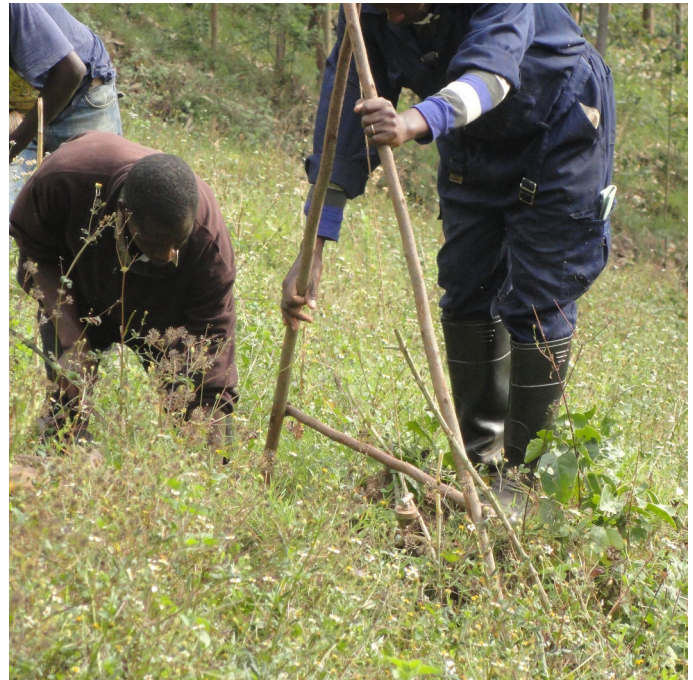
Use of the 'A-frame' to set out the soil and water conservation channels (Kenneth Twinamasiko)
