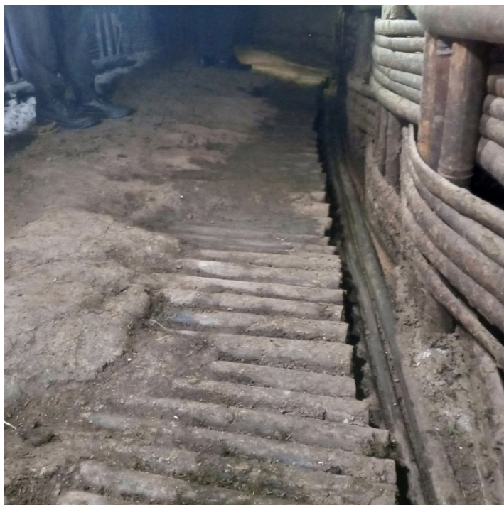
The floor of the cattle stall drains the urine straight to the collection chamber set outside the house. (Gerba Leta)
