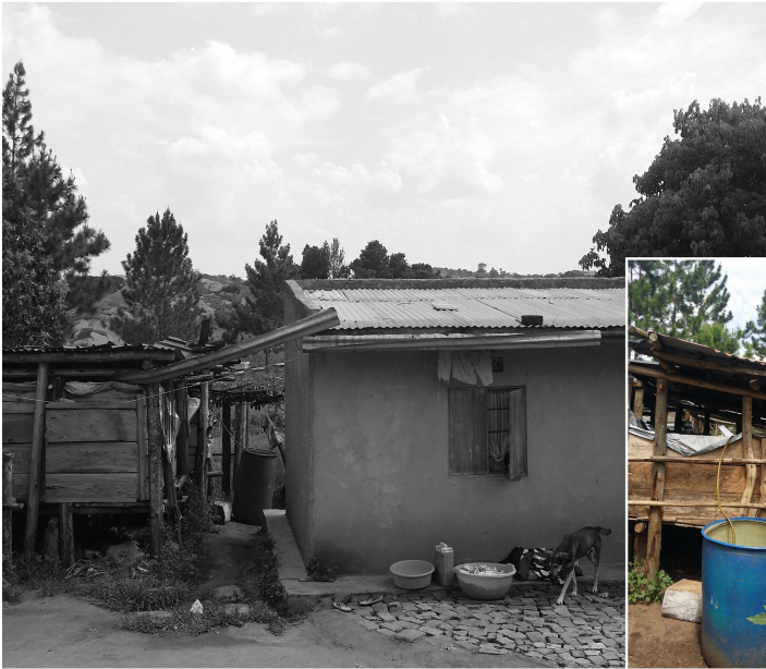
Front view of the rain-water harvest reservoir structure. (Aine Amon)
