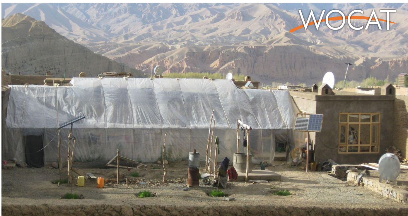
Passive Solar House belonging to Barat Ali for house warming during winter (SLMP (HELVETAS Swiss Intercooperation Afghanistan))
