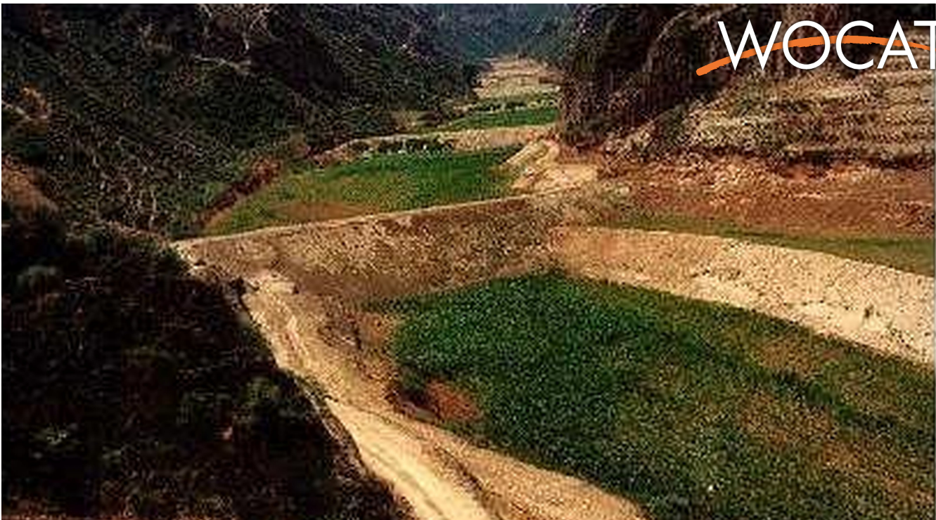
Construction of auto-flowing slurry dam in the gully (LIU Baoyuan (Beijing, China))
