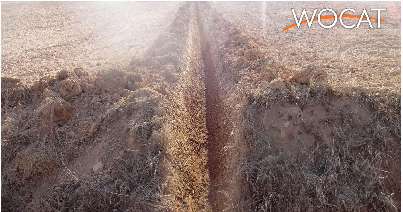
Drainage ditch constructed in a field with a problem of drainage and high calcium carbonate content. (Daniel Danano Dale)
