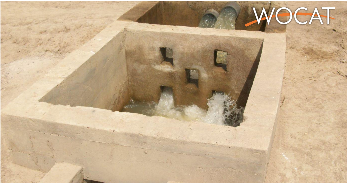
Delivery basin and energy dissipation structure (Minamba Traore, IICEM)
