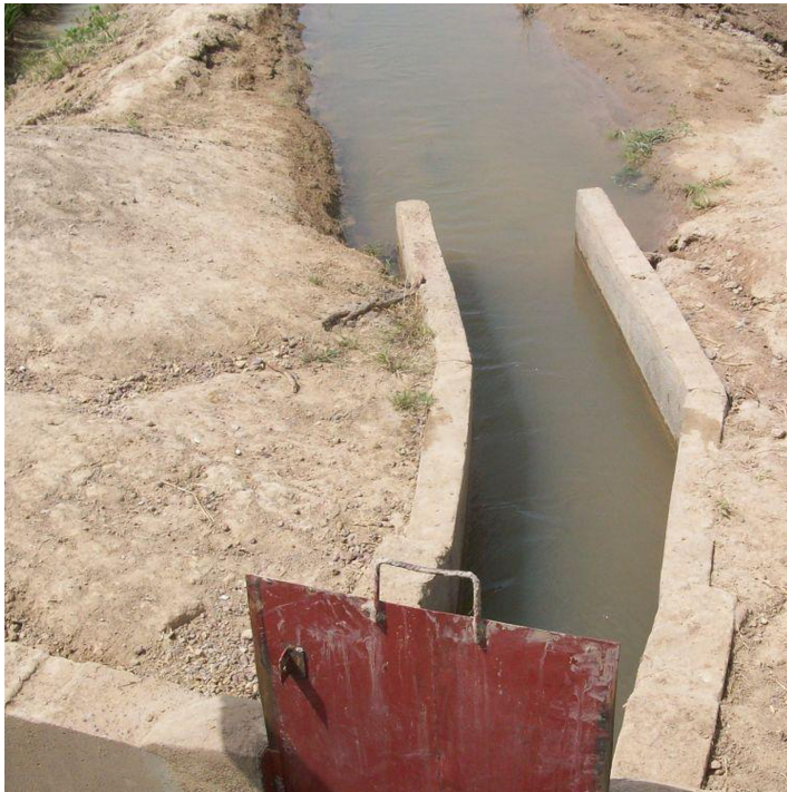
Turnout from a main canal into a secondary canal (Minamba Traore, IICEM)
