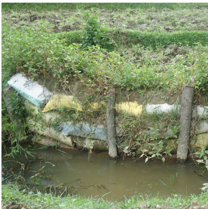
A retaining wall built using earth-filled sacks and bamboo posts. Tree seedlings and local grasses are planted on top of the retaining wall to help stabilize it. (Sabita Aryal Khanna)
