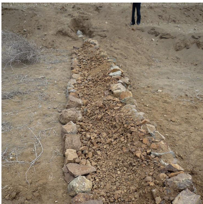
Building of a stone wall check dam. (Simon Bach (CDE, Bern, Switzerland))
