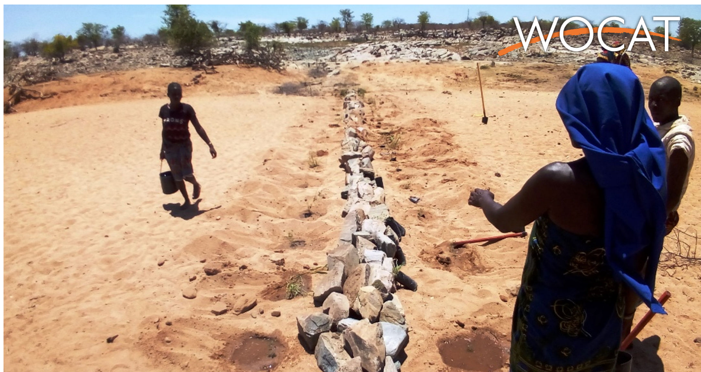
Members of the Tchicolongilo Community building and planting a 'Leaky weir' near the Caungo Natural Springs. (Projecto RETESA)
