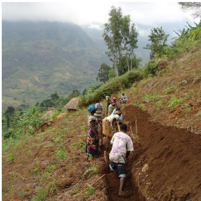
Farmers excavating Fanya juu terraces to reduce run off and improve crop production (Erasto Massoro)
