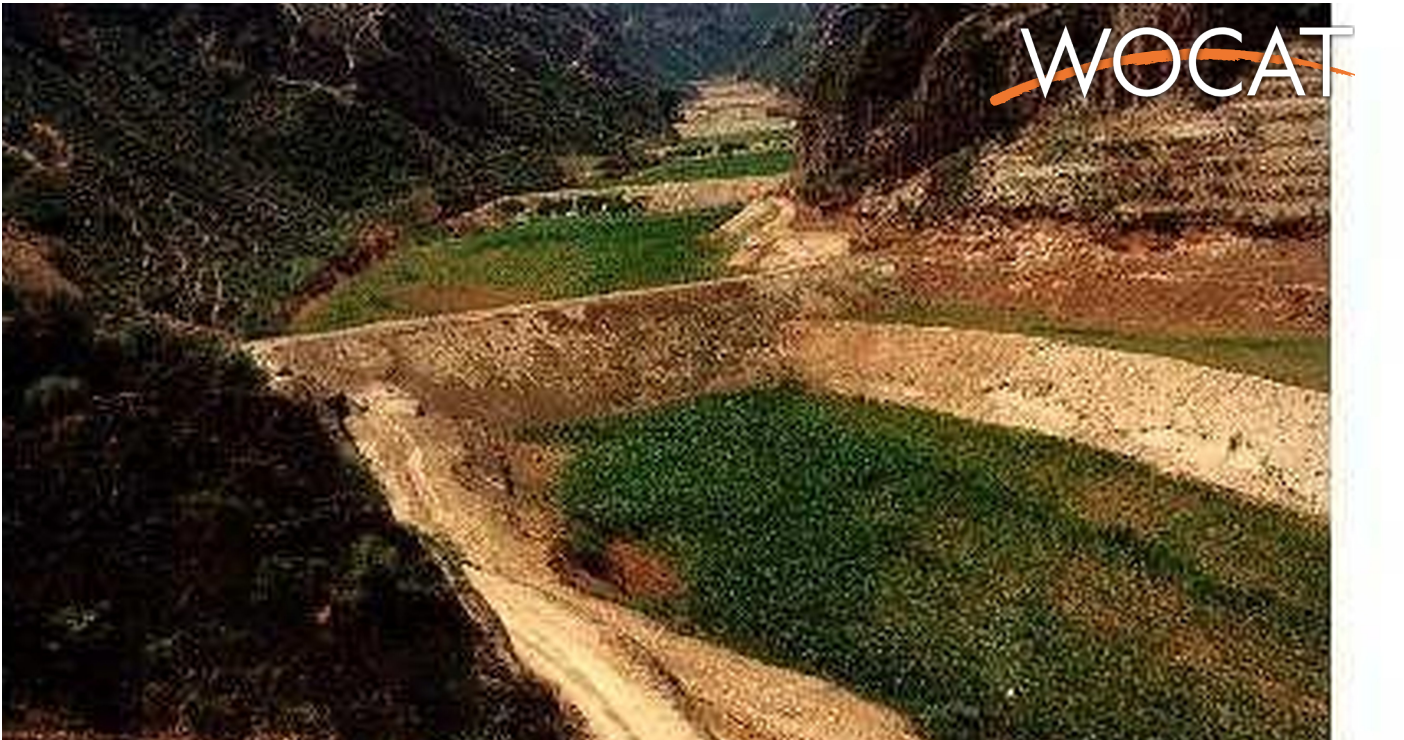
Construction of auto-flowing slurry dam in the gully (LIU Baoyuan (Beijing, China))
