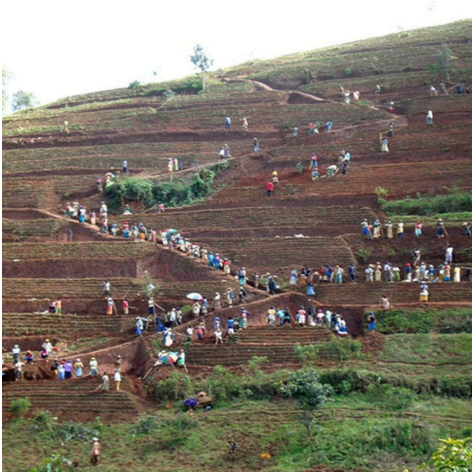
Radical terraces under development by communal group work (Umuganda) (Kagabo Desire and Ngenzi Guy (RAB))
