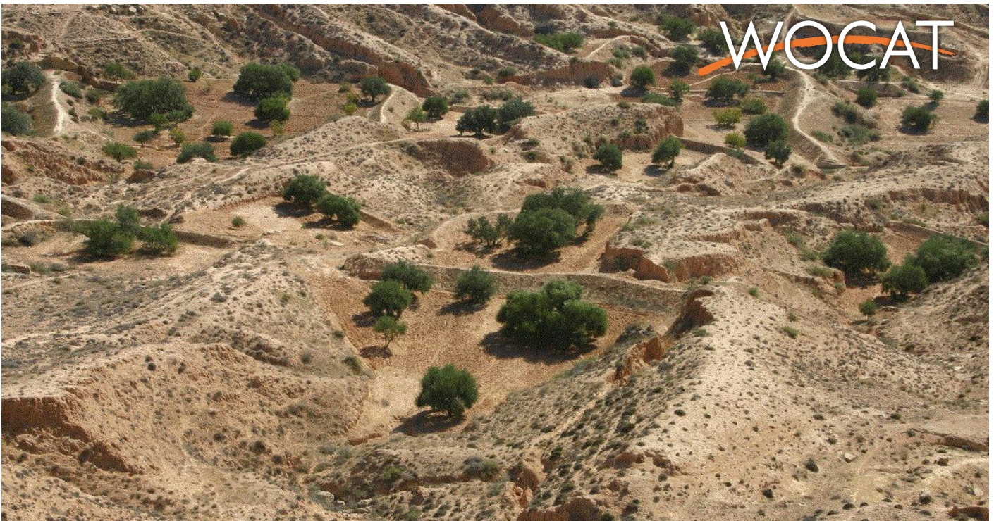
Jessour is the plural of a Jessr which is the hydraulic unit comprising a dyke, spillway, terrace (cropping area: fruit trees and annuals), and impluvium (runoff catchment area) (van Delden H.)
