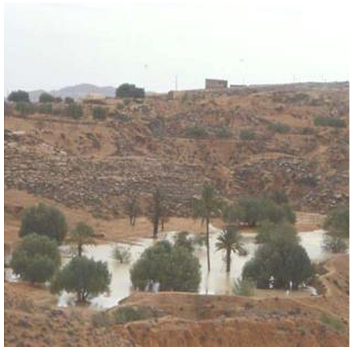
Jessour is an ancient runoff water harvesting technique widely practiced in the arid highlands of southern Tunisia. (Ouessar M. (Medenine, TUNISIA))
