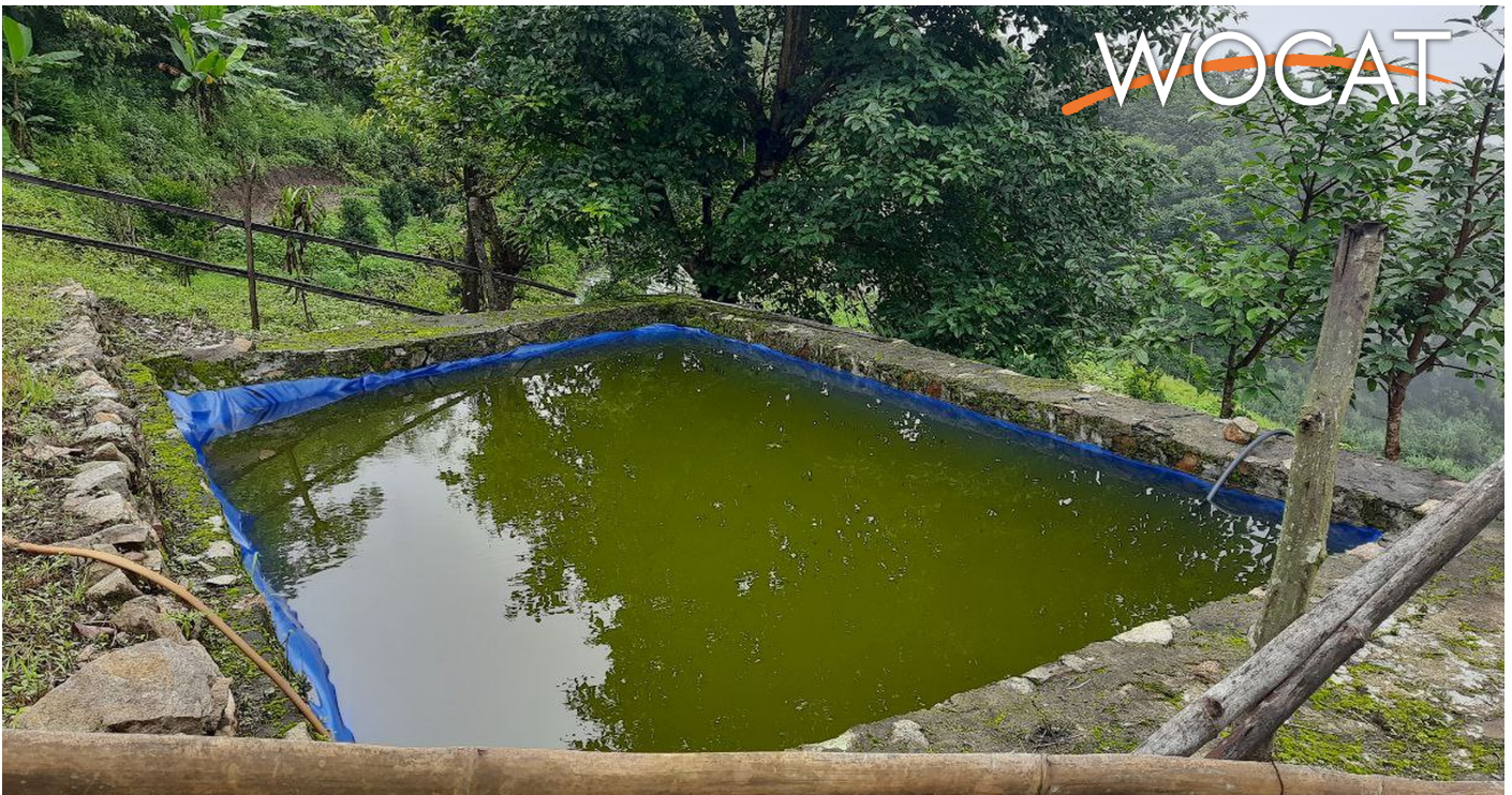
Low-cost plastic-lined water harvesting pond (Thinley Penjor Dorji)
