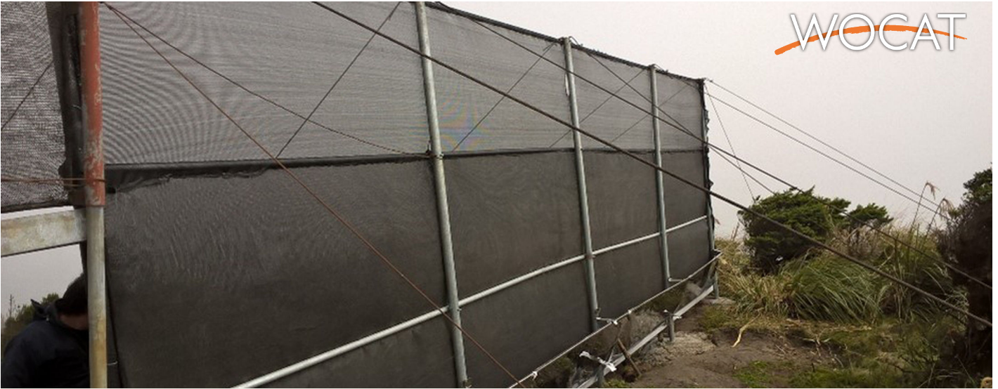
Fog water capture system (Carol Tapia)
