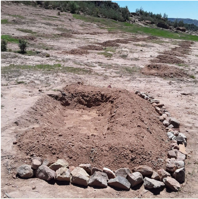
Full details of a constructed infiltration pit. Stone layering is used to support the walls of the pits and to discourage erosion (Koetlisi Koetlisi)
