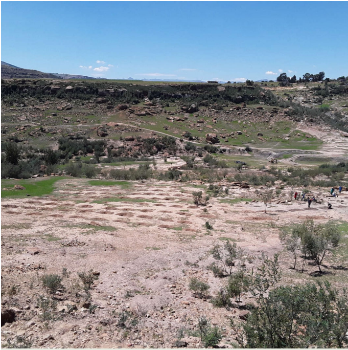
Overview of area constructed with infiltration pits in one of the catchments, Likhakeng Ha-Mahlomola Leribe (Matoka Moshoeshoe)
