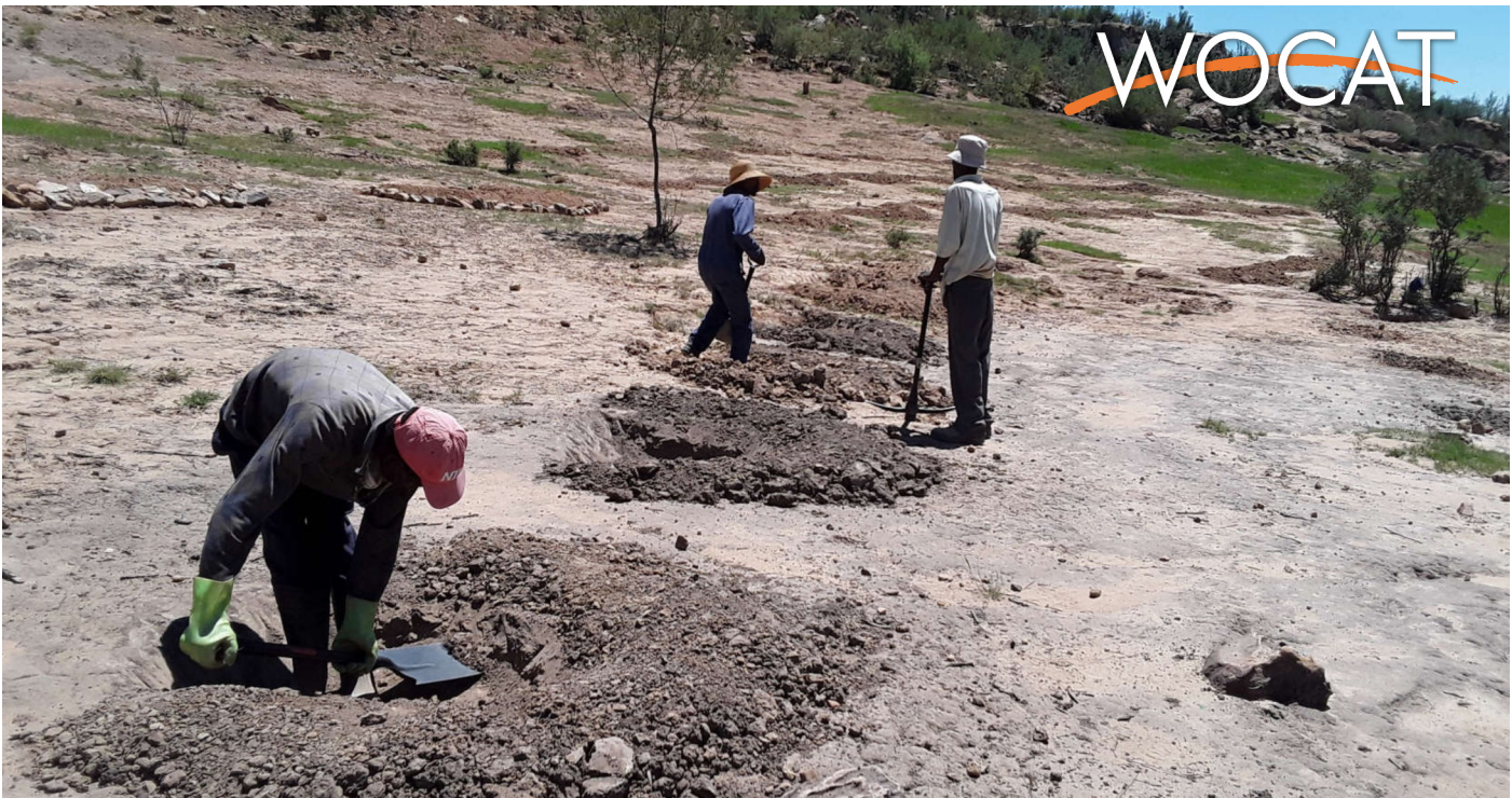
Infiltration pits constructed on bare land to improve land cover, land productivity and soil organic carbon. Leribe district. (Koetlisi Koetlisi)
