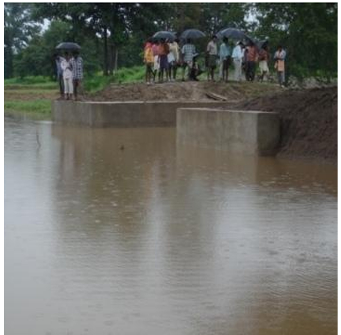
Up Stream of the Diversion Weir
