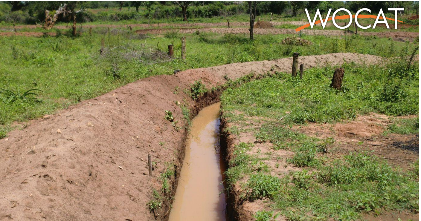
A constructed retention ditch in lower Mbeere South District (Paul Kahiga (P.O.Box 8444-00300 Nairobi))
