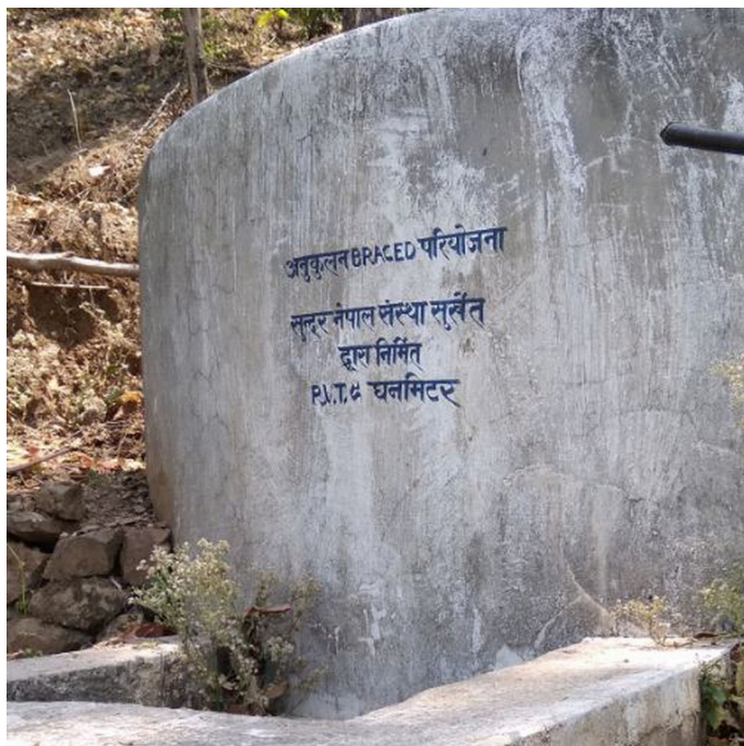
Ghaito / Ferro-Cement Tank, Saajhpani, 9000L (Jhuna Kattel)
