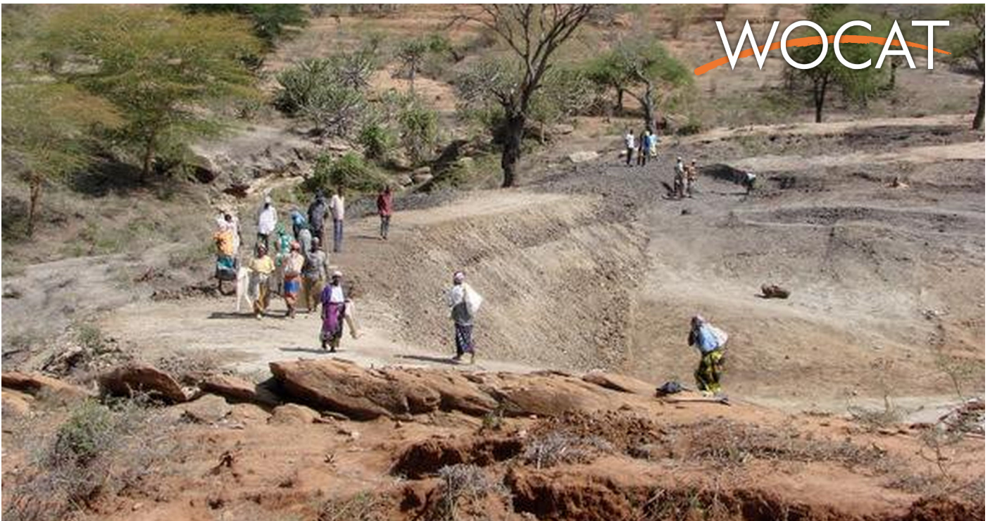
Manual construction of a small dam requires community action: soil is transported in bags, piled up and compacted layer by layer (Maimbo Malesu)
