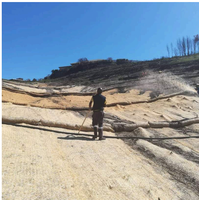
Application of hydroseeding after construction of the fibre rolls and erosion blankets (J Buckle)
