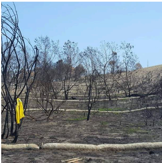
All loose burnt material must be removed prior to the construction of the fibre rolls and placement of the erosion control blankets (J Buckle)
