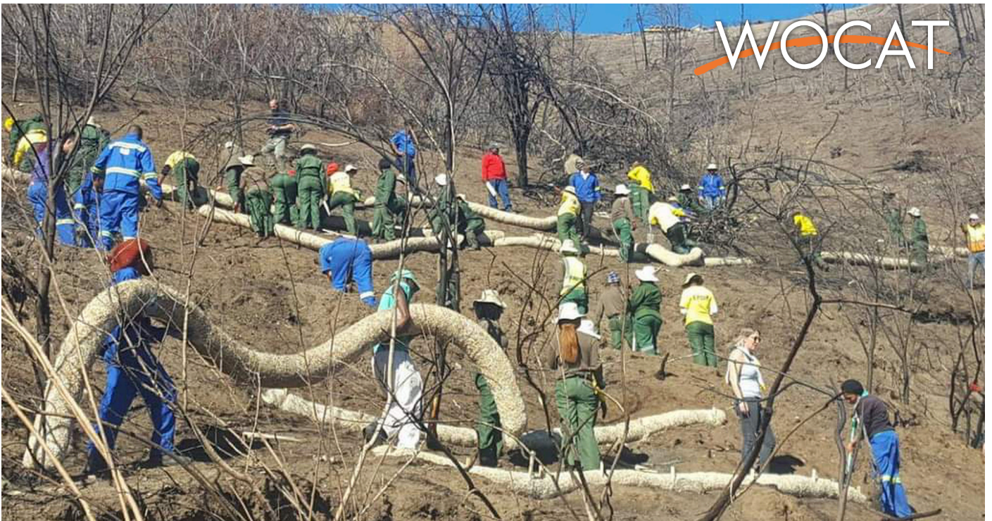
The introduction of sediment retention fibre rolls (SRFR) and erosion blankets to stabilise slopes after vegetation cover was destroyed by fire (J Buckle)
