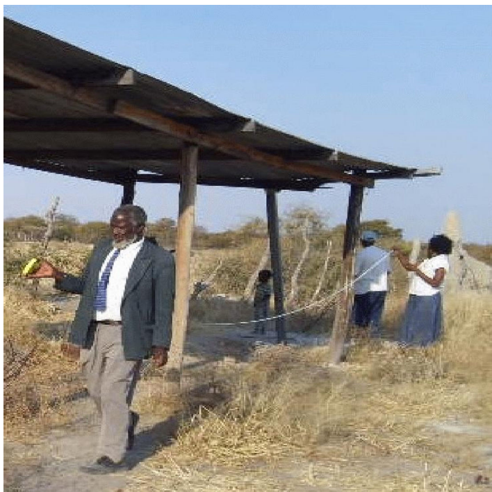
Taking dimensions for a rainwater system in Mopipi lands ((M. Moemedi))
