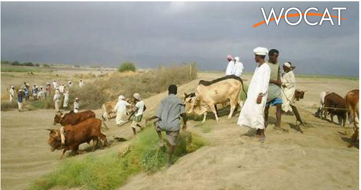
Social organisation and community action are prerequisites for spate irrigation systems: construction of an agim in a dry river bed (IFAD)
