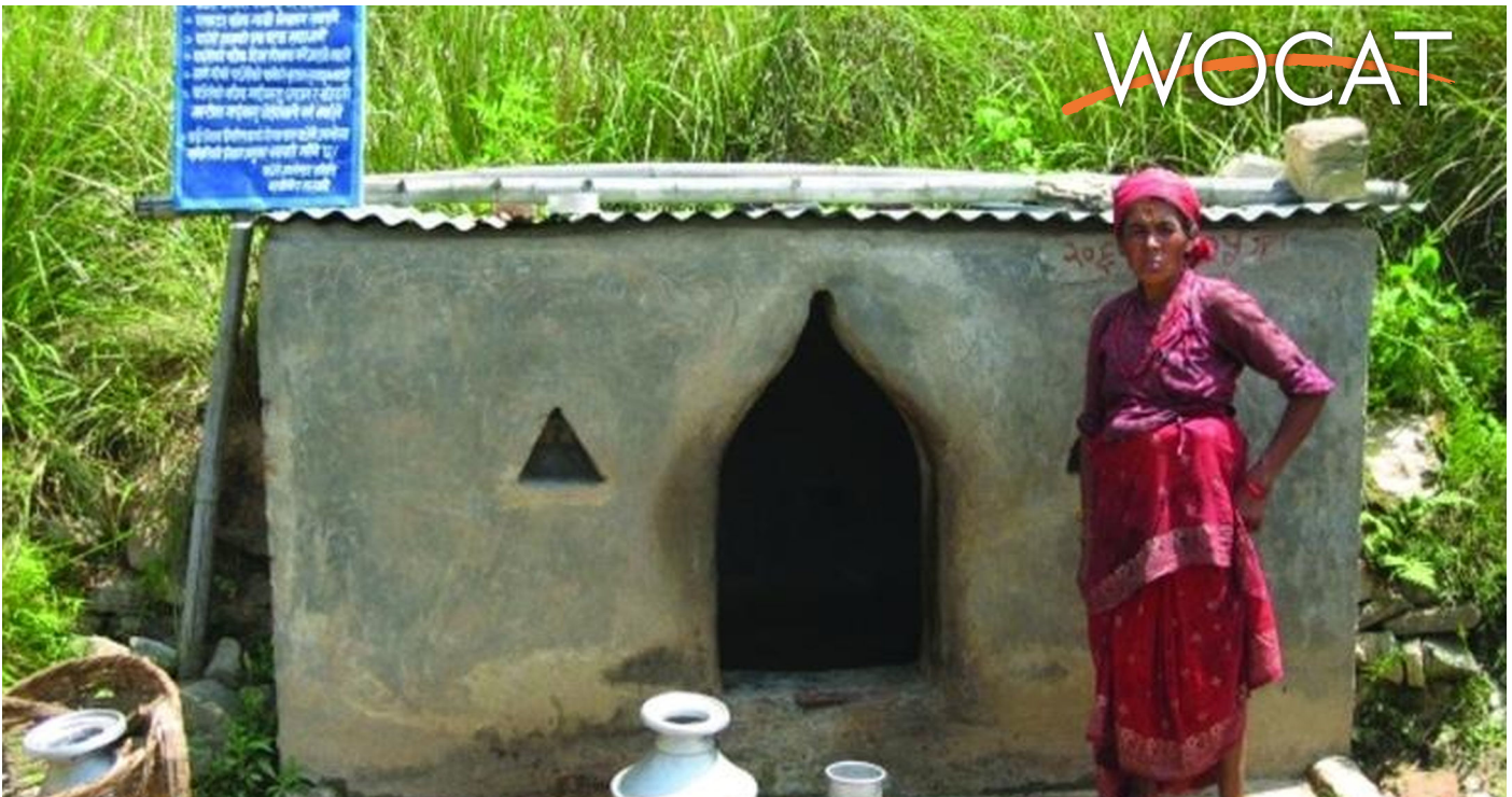
Brick-cement walled spring box (check dams were established to prevent surface water flowing directly into the spring and (Sanjeev Bhuchar)
