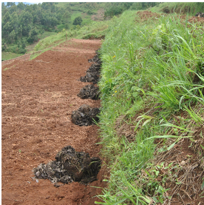
Newly constructed bench terraces planted with starria grass on the riser for stabilisation (Kenneth Twinamasiko)
