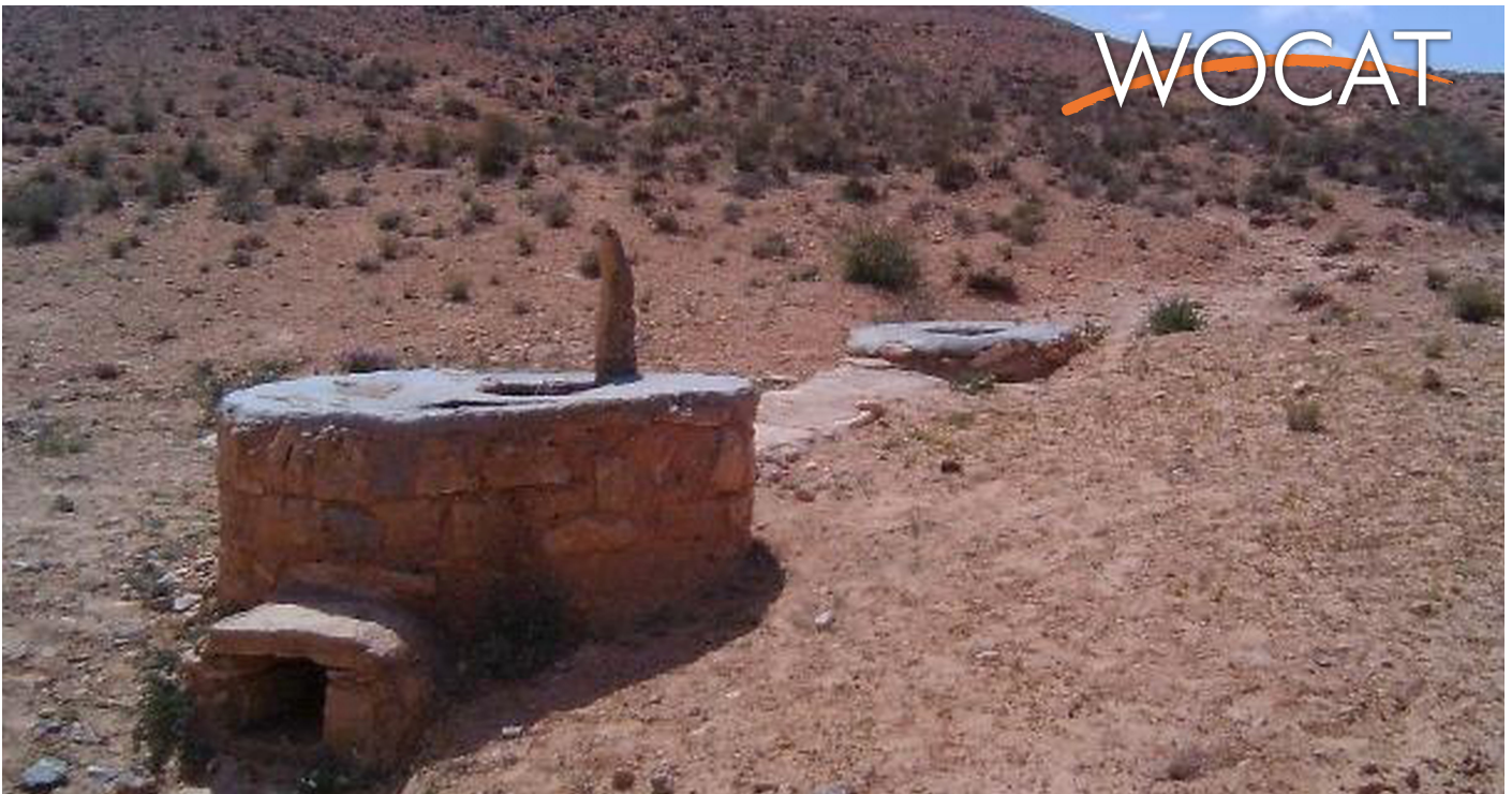
Different components of a cistern (majen/majel): the impluvium (collection area), the decantation basin, the main reservoir, and the outlet. (Ouessar M. (Medenine, Tunisia))
