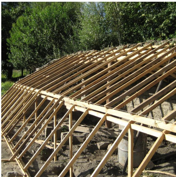
South-facing side of a solar greenhouse during construction process before the cellophane layer was put in place (MSDSP Khorog)
