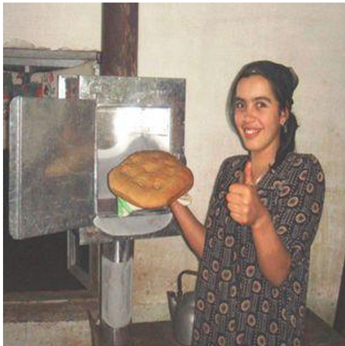
Heat exchanger installed on chimney to retain heat and for cooking. (Firuza Hafizova (40, Shamsiddin Shohin, app.32, Kulob city))
