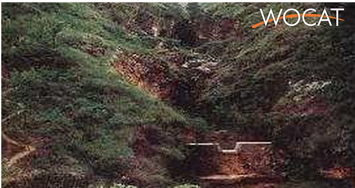
Check dams in a gully of the Loess Plateau.
